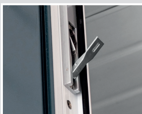
Flush bolt to lock the inactive leaf (top and bottom)
